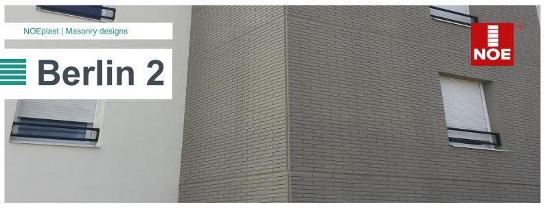
Concrete surfaces made with this textured formliner reproduce the appearance of sand-lime block walls with a unit size of 240 x 52 mm. The concrete walls have the advantage that they are constructed in one pour and therefore completed much quicker.
