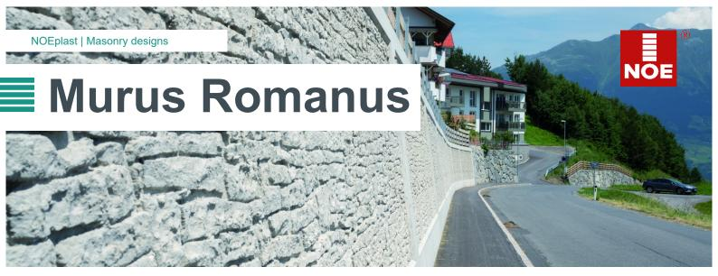
An extremely popular texture because it creates the impression of a roughly coursed wall made out of broken natural stone. The natural colour of the concrete alone is often sufficient to create a convincing appearance.
