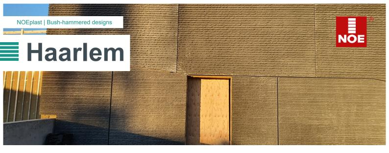
The Haarlem textured formliner is one of the bush-hammered designs. In contrast to the Antwerpen II, the ribs on the Harlem differ in size.
