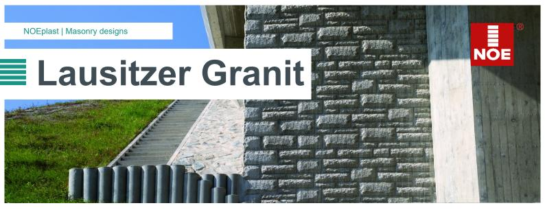
Hewn granite stones of various formats were the model for the Lausitzer Granit textured formliner. The availability of corner textured formliners and the interlocking (toothed) longitudinal butt joints between formliners make the Lausitzer Granit perfect for a wide range of applications.
