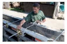
**Tying without grid patterns** by using tying claws above the formwork.
