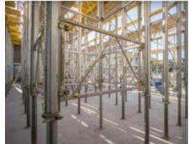
NOEprop is compatible with almost all deck systems The horizontally or vertically fitted support frames allow flexible arrangement of the props
