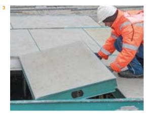
Earlier stripping, as props directly support the concrete slab
