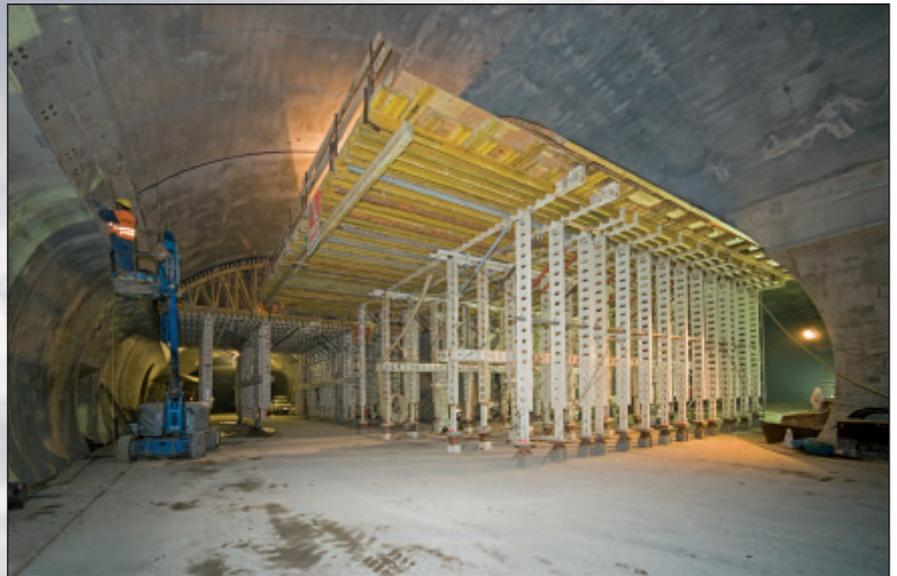
Use as centring soffit formwork
