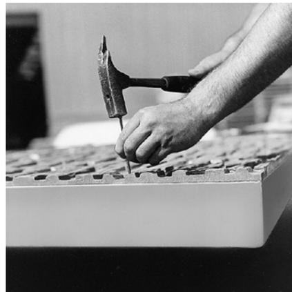
Nail or screw down the formliner at the corners. Screw clamps can be used to hold down the formliner in the case of steel formwork (see photos). Ensure that the whole area has been pressed down.
