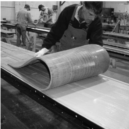
After applying the adhesive to the whole of the back of the NOEplast textured formliner, place the formliner down on its long edge and unroll it onto the formwork substrate. Press the formliner into place without trapping any air. If necessary, weigh down the corners and edges.
