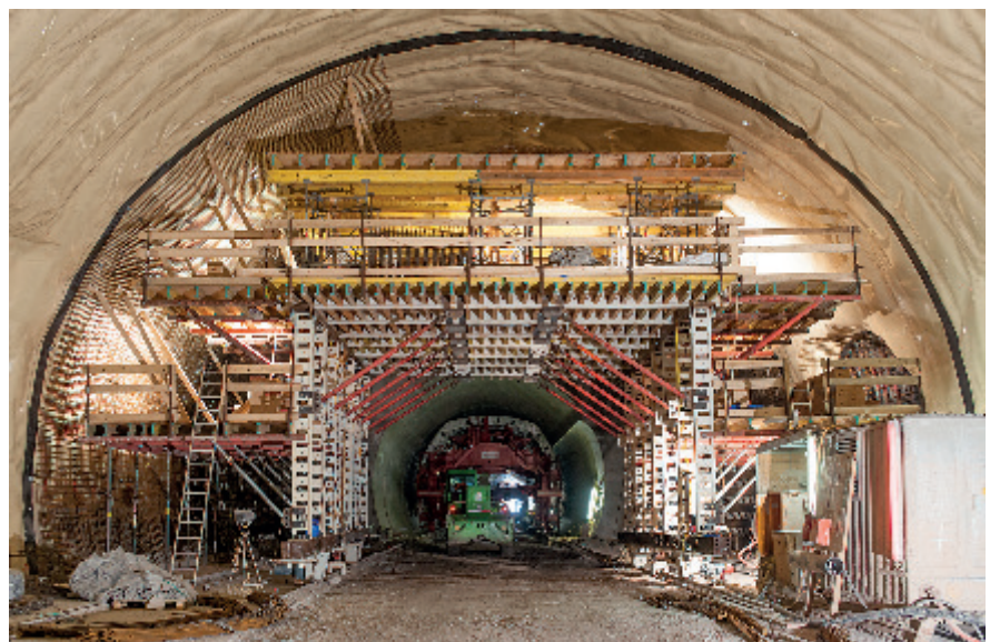
Two tunnel formwork carriages, traditional tunnelling construction, reinforcement carriage
