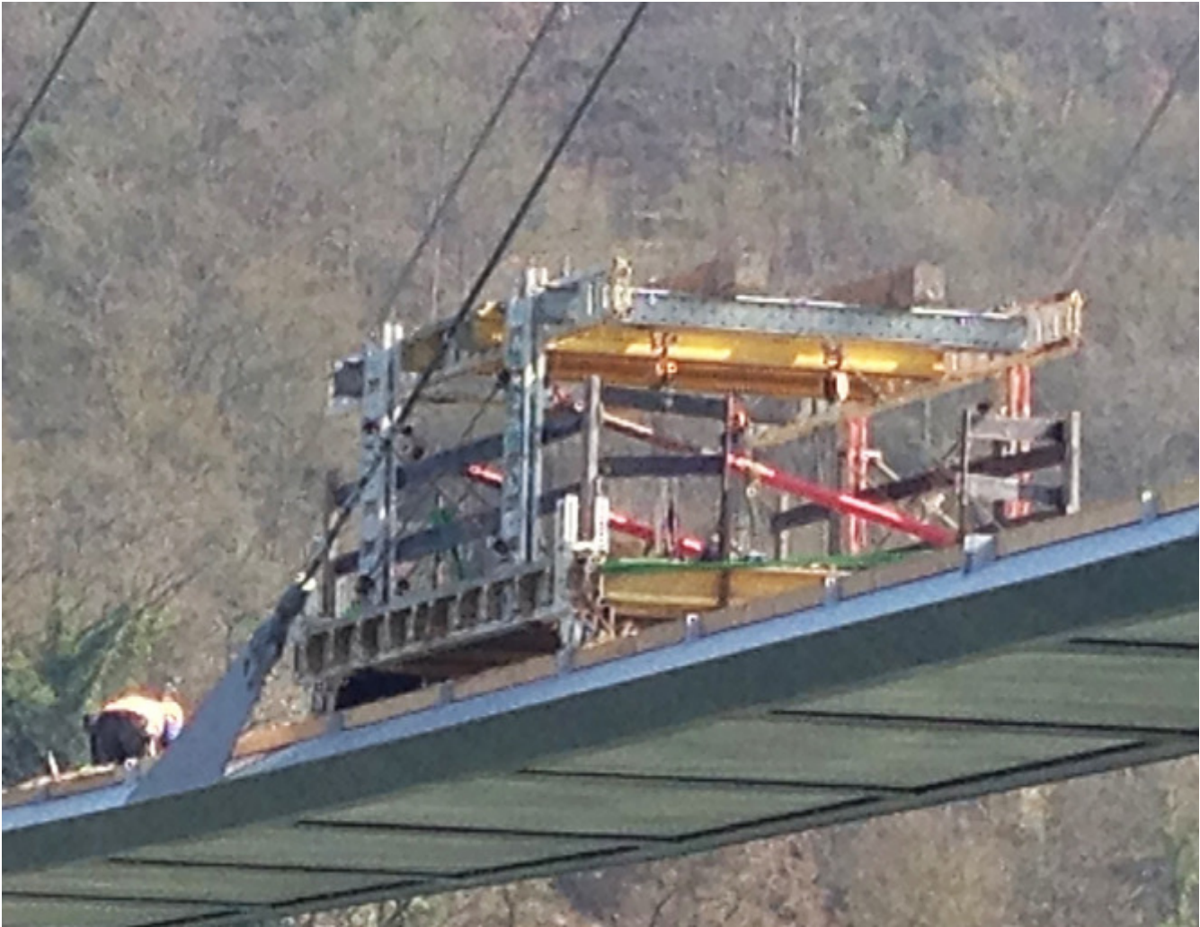
Transport carriage for precast concrete units
