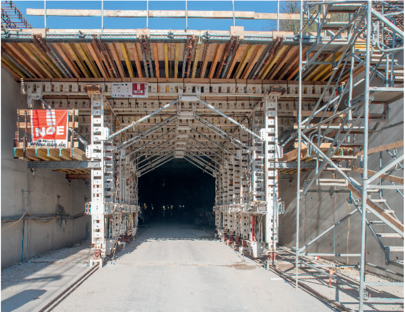
Two tunnel formwork carriages, traditional tunnelling construction, reinforcement carriage
