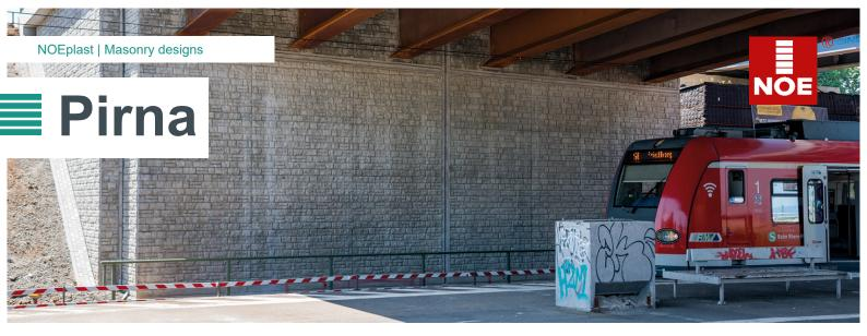
An irregularly coursed natural stone masonry wall. Pirna is often used on bridge abutments and piers.
