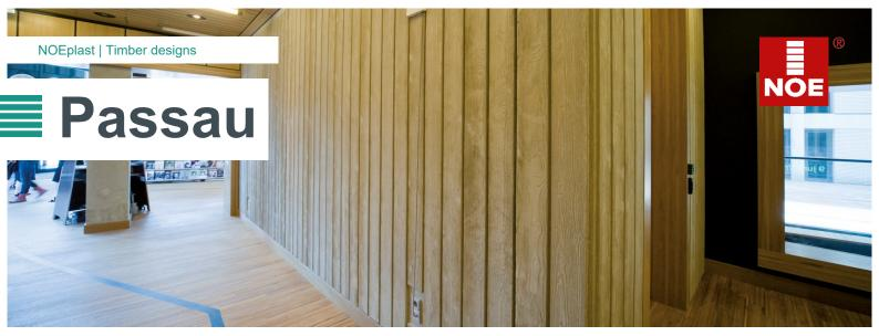
The model for the Passau textured formliner was an arrangement of traditional 182 mm wide tongue and groove boards with a 22 mm wide groove. The boards were brushed to bring out the detail in the appearance of the concrete.
