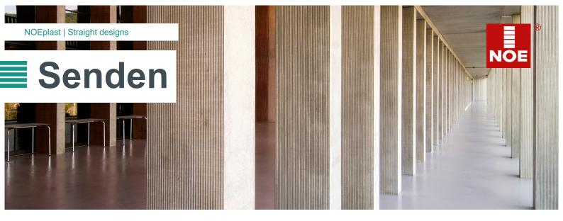
A soft ribbed texture, the ribs being rounded and placed closely adjacent to one another.
