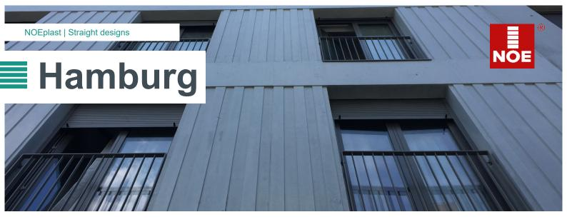
This textured formliner imitates the texture of smooth, painted boards. Alternate boards are at different heights.
