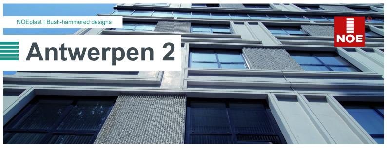
A concrete panel with the trapezoidal relief Antwerpen was used as the original model for the Antwerpen II. The trapezoid is struck off using a hammer, which creates irregular broken edges.
