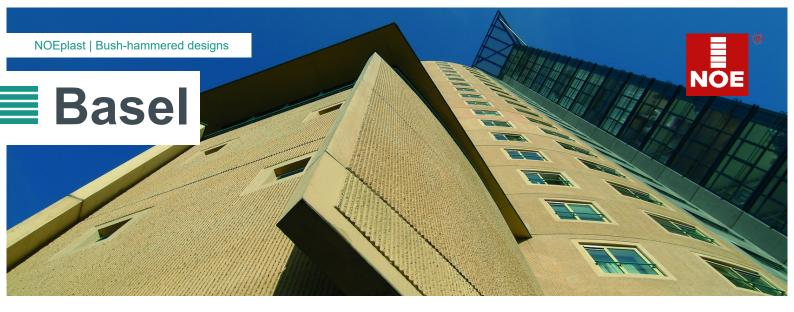
A concrete panel with circular ribs similar to the Genf textured formliner was used as a model for the Basel. The ribs are broken off with a hammer to produce irregular fractured edges.
