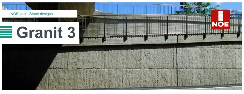
This textured formliner gives the concrete the appearance of a large granite panel with a coarsely hewn surface. Unlike with Granit II, the formwork designer does not have to consider the direction of the texture.
