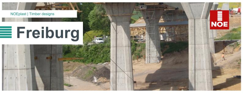
Chamfers have been deliberately omitted to create a smooth transition between the rough-sawn boards. At the end of the 10 m long formliners, the ends of the boards are irregularly stepped and interlock so that the end butt joints are hardly noticeable. This creates the appearance of a consistent timber texture covering the whole surface.
