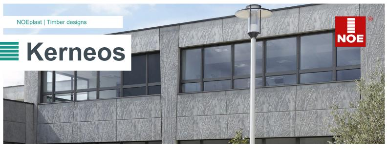
This bamboo-like plant relief is best used over the full 7.95 m height of the textured formliner. However, parts of the Kerneos can also be used to create a nature-themed surface.
